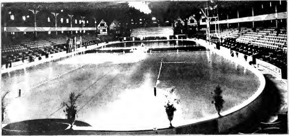
FIG. 31. ON JUNE 18 THE POOL WAS OPENED, HAVING BEEN COMPLETED IN 47 CALENDAR DAYS OR 39 WORKING DAYS
